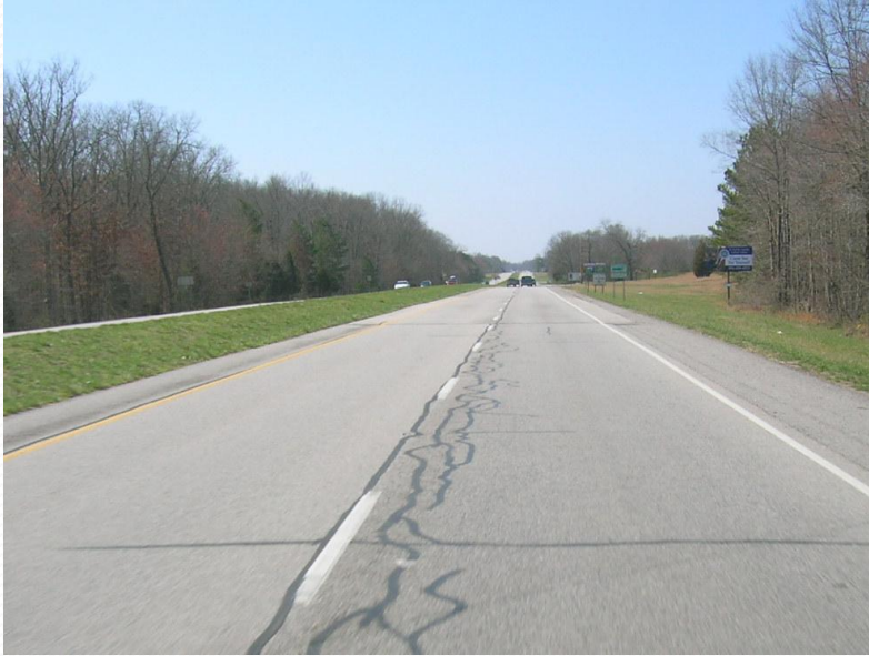
Crack filling/ sealing
